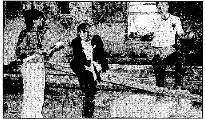
Left to right, architects Scott Crow and Norma DeCamp Burns of Burnstudio check the progress of construction with Grover Edwards of Edwards Construction
