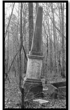
Nathaniel and Rachel Jones graves in former state of disrepair (courtesy NC Department of Archives & History, via Anne Kratzer)
