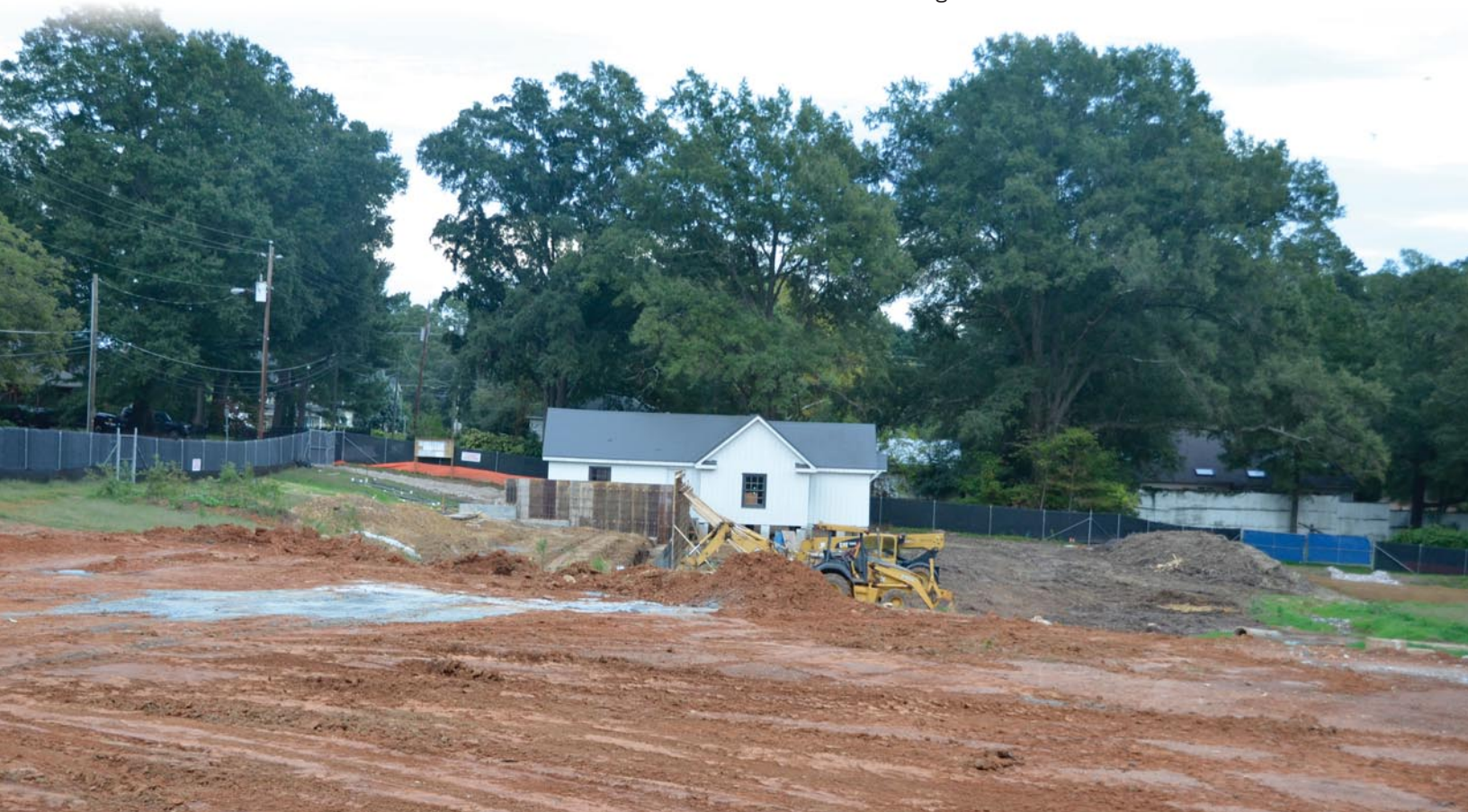
Below: The Waldo house sits at the construction site, awaiting renovation.
